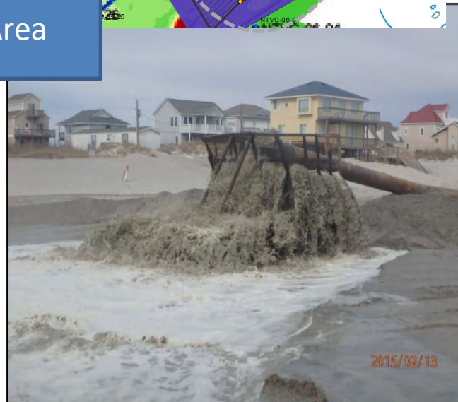
Figure 35. Rock box installed during dredging operations.
