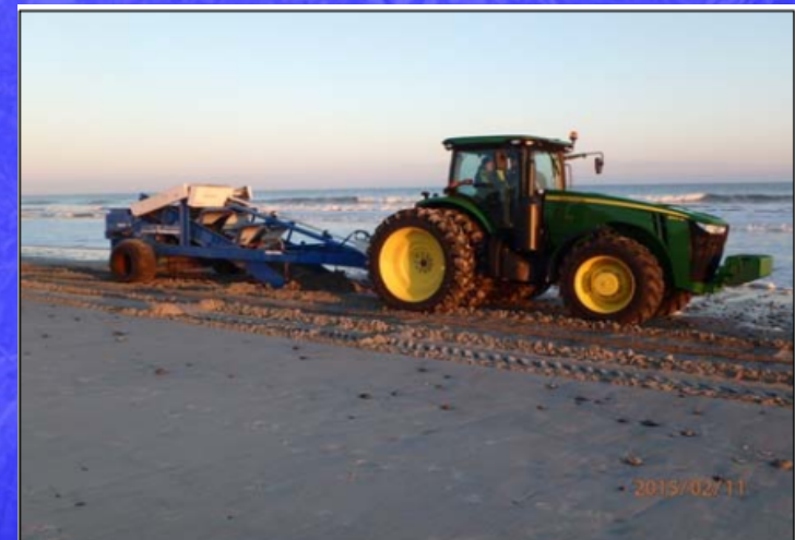
Photo 2. The rock picker was dragged behind a tractor along the beach fill area to remove rocks between Sta. 755+00 to 750+00.
